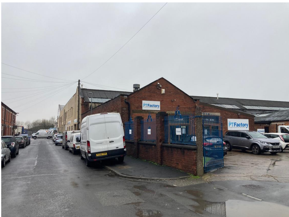
Photo 4: View westward along Holland Street West, from junction with Derby Street, and of existing yard entrance
