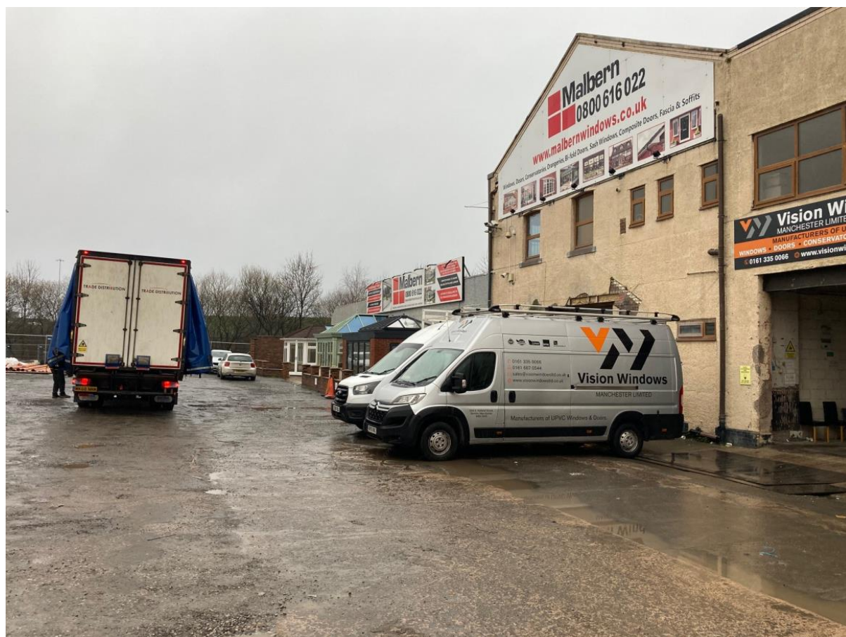
Photo 2: View of existing building and adjacent yard area
